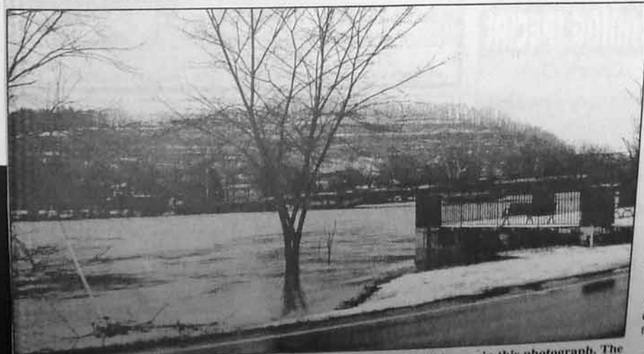
High levels of water can be seen rushing under the bridge in Alderson in this photograph. The water ultimately crested there at 3.2 feet above flood stage early Sunday morning. Debbie Dunbar photo
